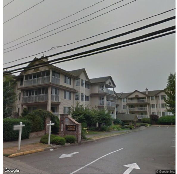
Strata Apartment - Frame
