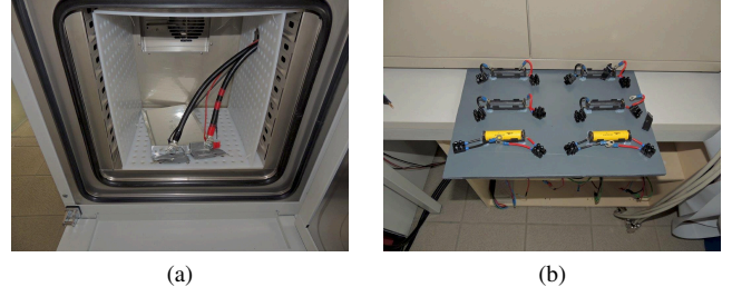
Fig. 10. Experimental setup. (a) Li-Titanate cell in temperature chamber (a), and (b) two LiFePO 4 cells connected to the power brackets.
