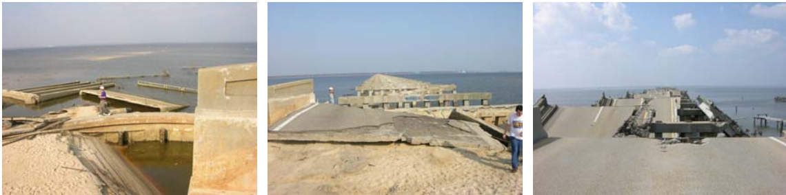
Figure 4 Traffic bridge from Bay St. Louis - piers in the center, and the roadway, flipped over, to the left - the right photo is from the East end
