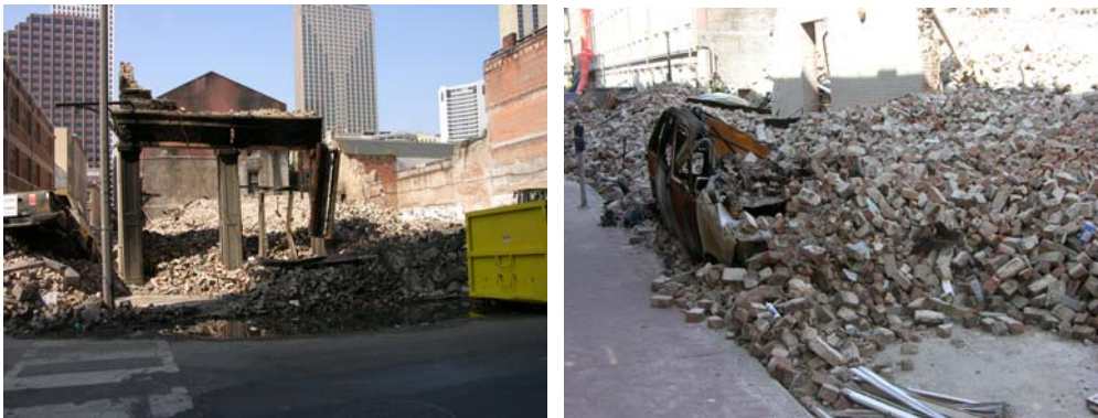
Figure 9 - Demolished brick building
